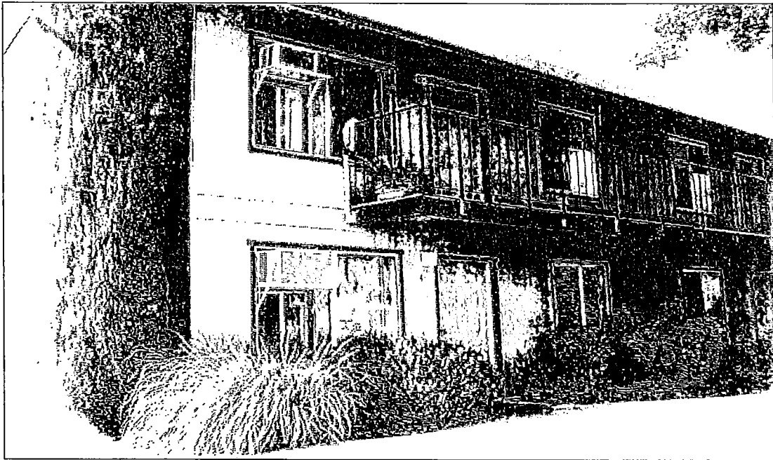
Figure B-5 Location: 842 F Street
