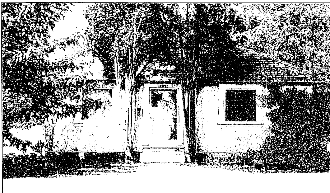
Figure B-2 Location: 2137 F Street
