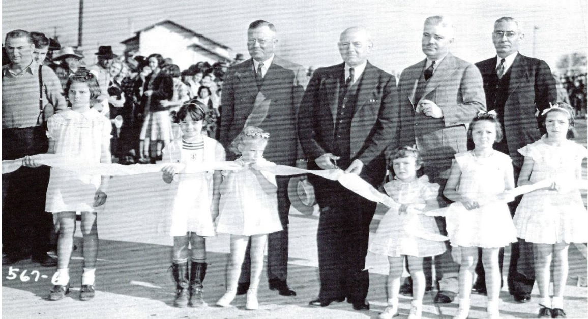
Opening of Underpass and Freeway through Livingston—1939
