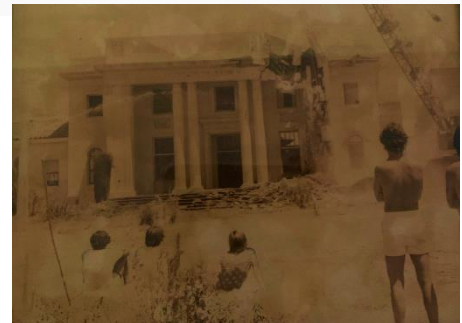
1977 Demolition of Livingston High school
