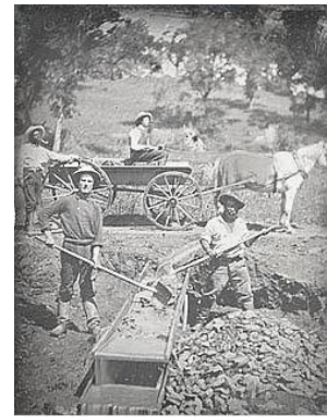
1852 miners in California work their "long tom" to separate gold from gravel.
